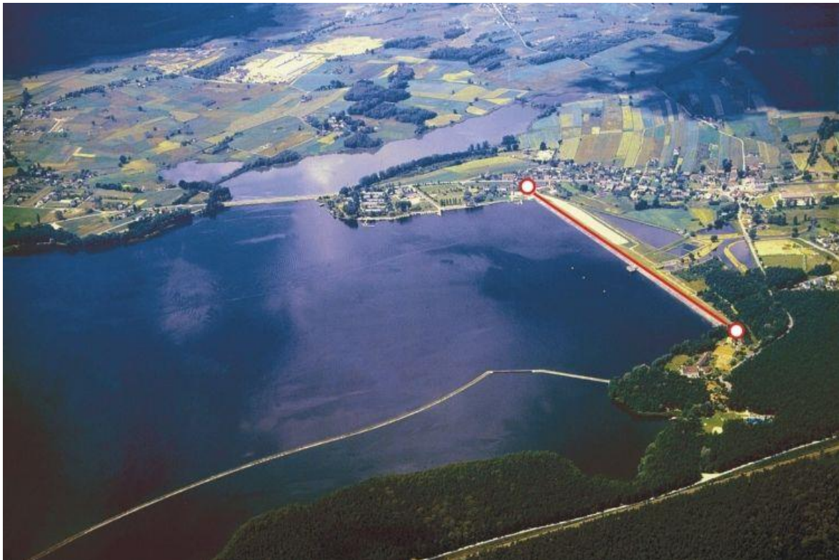
Fig.1 The front dam of the reservoir in Rybnik, the southern Poland. This reservoir supports large coal plant and helps to mitigate floods. The survey were 800 m long along the crust of the dam for seismic, end extended to 3D survey for ERT and GPR measurements.
